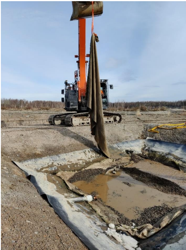
Figure 12. Mats renewal process on going (Feasib 10.5.2022).
