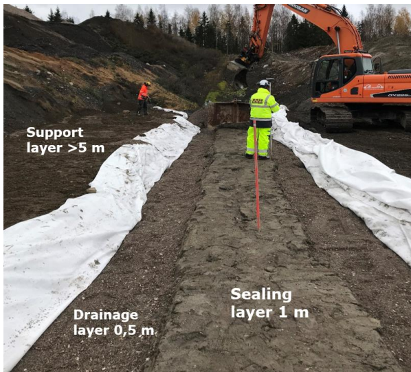
Figure 9. Vertical sealing barrier.
